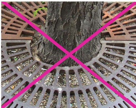
Poor size selection for the tree opening results in an unfinished look, significantly crowds the tree, and impairs proper tree growth.
